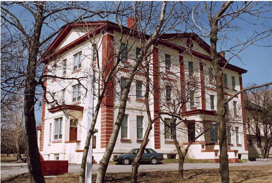
The now closed and demolished Mount Cashel Orphanage in St. John's, Nfld. Register file photo
